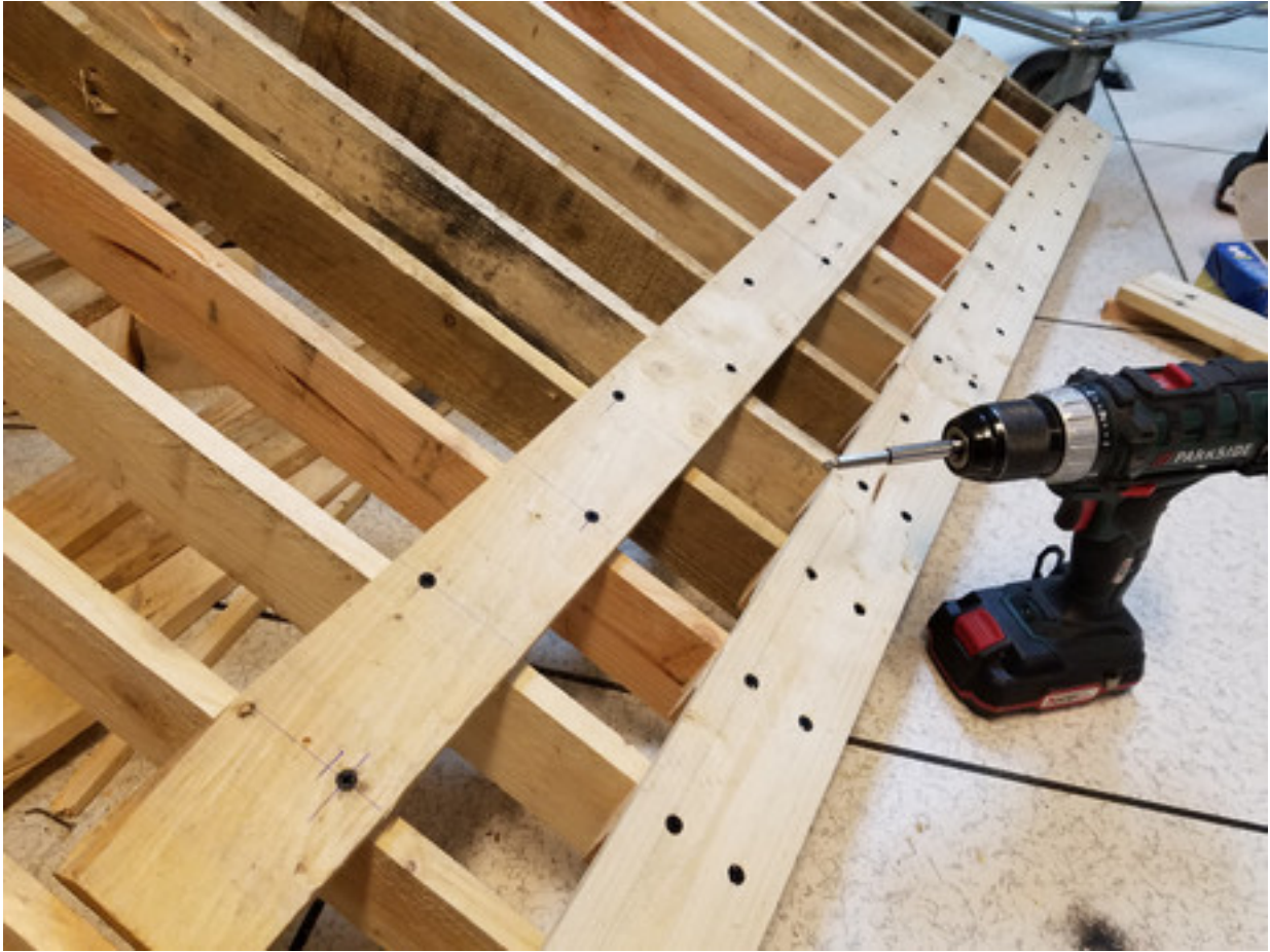
FIGURE 5.39. – planche de support vissée
