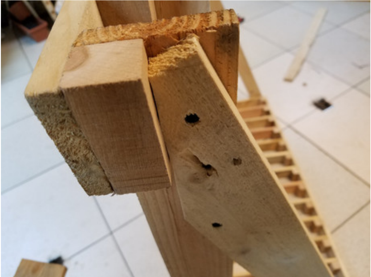
FIGURE 5.36. – planche diagonale vissée
